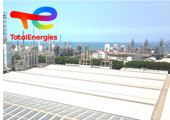
4,800m 2 of Solar Panels reducing up to 644 tons per year of CO 2 emissions
