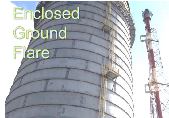
EGF leaves no air discharge, reduces noise, eliminates heat & smoke
