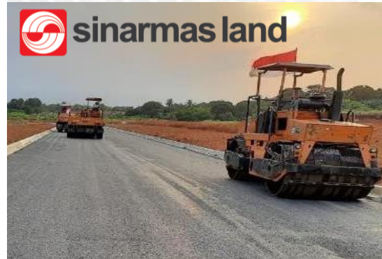
Application of 15,518 m 2 of plastic asphalt in BSD City with PT Sinarmas Land
